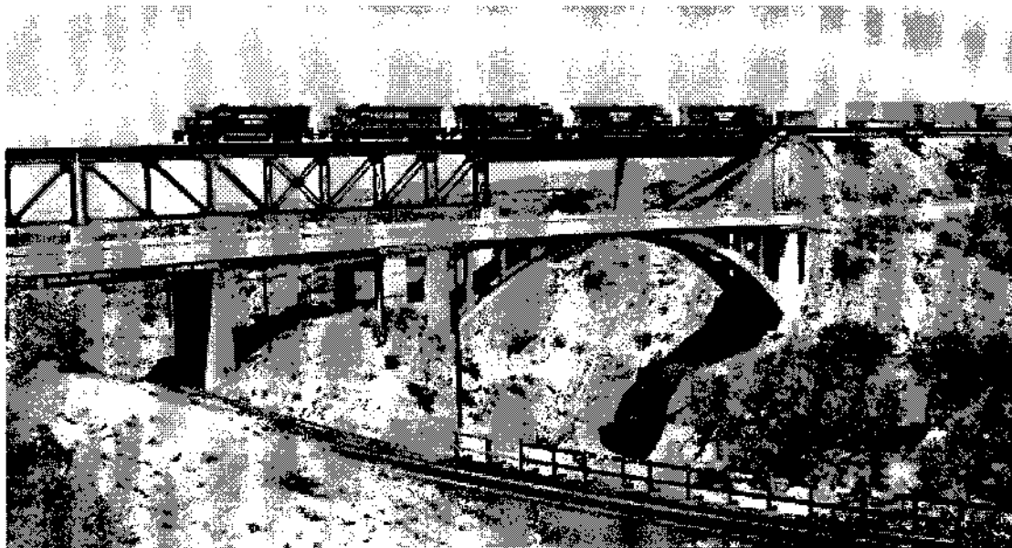
Fast trains such as this one demand high standards of maintenance of motive power and equipment well as track and signal systems.
